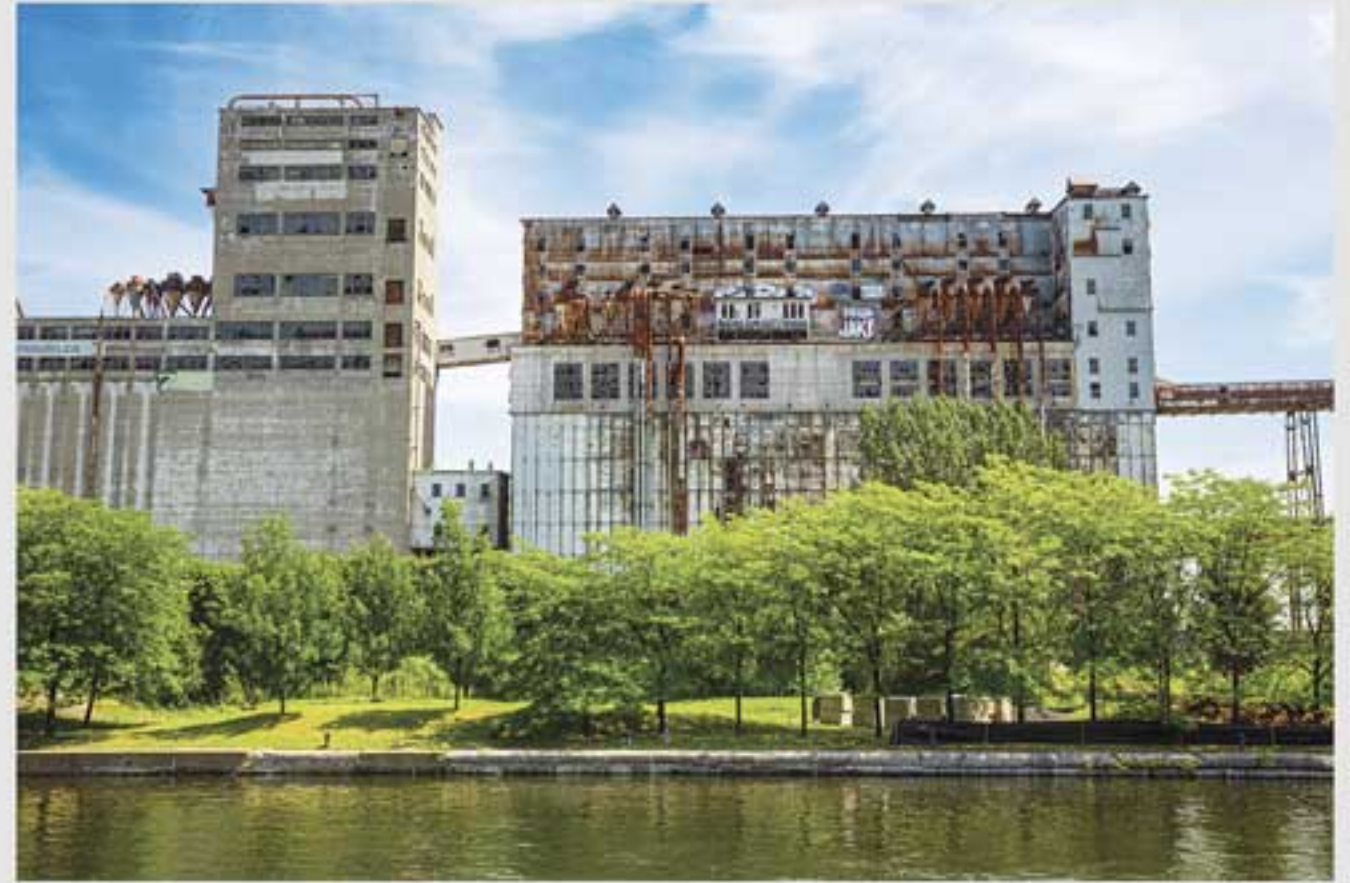
M4- Silo No.5
